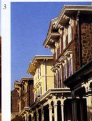
③ A terrace/row in the Italianate style, in Philadelphia, with roof pediments, elegant porches and ornate eave brackets. Italianate was probably the most prominent townhouse style from the 1850s to the 1880s. WT
