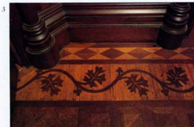
③ and ④ Two fine parquetry floors, in light and dark woods. NA
