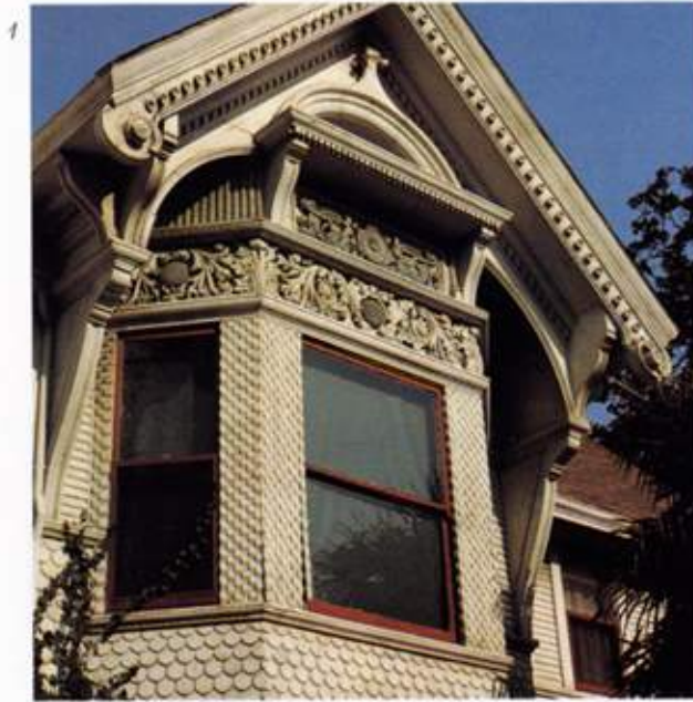
① A detail of a Los Angeles Queen Anne house of 1894, showing exuberant use of mass-produced millwork. JBE
