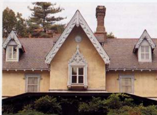
④ The Gothic Revival style is characterized by steeply pitched roofs, dormer windows, and a curvilinear "gingerbread" trim along the eaves and gable edges. Gothic was greatly popularized by the architectural writings of Andrew Jackson Downing (1815-52). In The Architecture of Country
