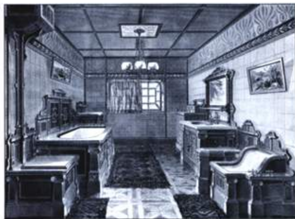
1 The early Victorian practice of enclosing plumbing fixtures in wooden cabinets built to match
