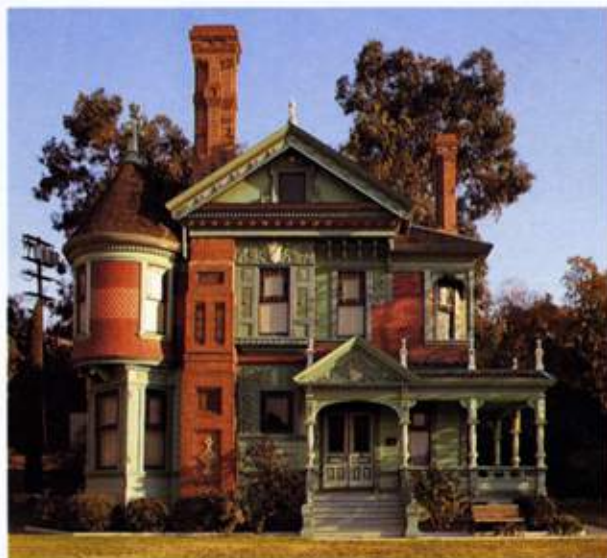
② The Hale House, Los Angeles, 1888: a sophisticated essay in wood and paint. This is an elaborate example of the Queen Anne style. The original colours have been restored, following meticulous paint research. HA
