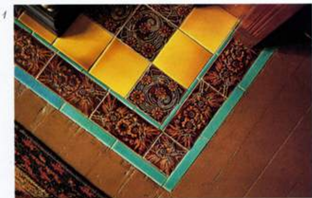
① A fireplace hearth of glazed tiles, set into the plain boards that were standard for the Victorian house. Glazed tiles
